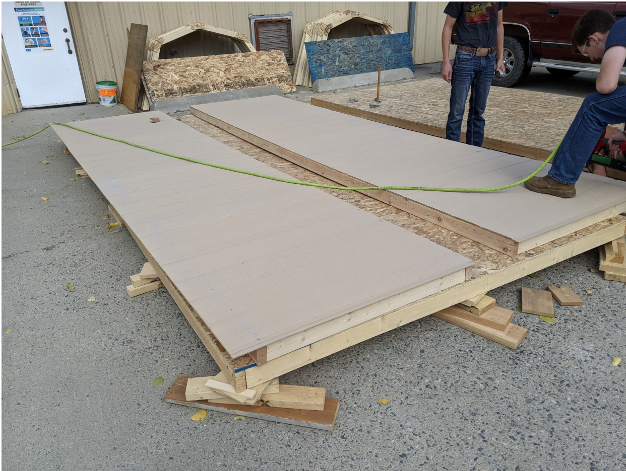
Carpentry: Capital High Students Building wall sections
