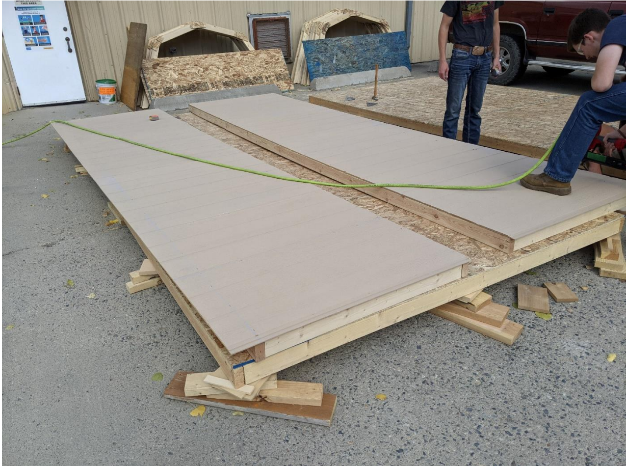
Carpentry: Capital High Students Building wall sections
