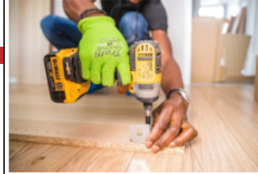
(Figure 1: New flooring and cabinets being installed in Classroom A1)
